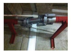
All expansion joints should be mounted in the axis direction between two pipes.
