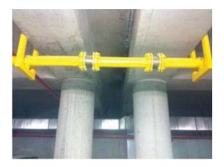
Of expansion joints with diameters over DN50 are to be used in natural gas pipelines, 2 standard axial expansion joints should be used, which should both be fixed at both sides of the line with welded connection.
