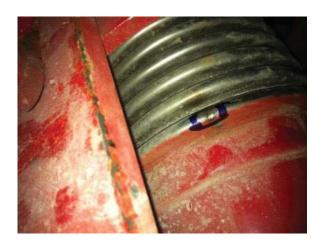
Care should be taken to avoid arc sparks falling onto the bellows during mounting.
