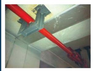
In case pipeline is close to ceiling, fixing can be done without using support brackets.
