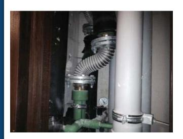
Heat expansion coefficients of plastic based aquatherm pipes are higher compared to steel pipes, therefore this should be observed when selecting the expansion joint and calculating expansion value. Natural omega should be applied in the first place in such lines.
