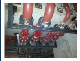
A sample fixed point. The pipe is fixed onto the main carrier profile at 3 different points. It is recommended that the main carrier profile is in box shape. A BOX PROFILE can be obtained by connecting 2 NPU profiles. NPU iron thickness must be selected by considering the load to be borne.
