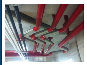
In V Flex applications, again there should be fixed points on both sides. F Flexes with same diameters are pushed inside each other for mounting. V Flex should be hung on the ceiling with a rod by using the fixing pin on the elbow, and L profile should be removed during installation.
