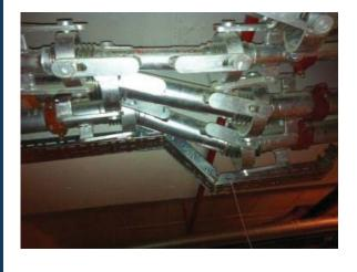
For expansion joint mounting on galvanized pipes, fixed points should be applied at a distance of L/2 of expansion joint length by taking special precautions.
