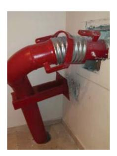
Fixed points should be created before and after elbows for expansion joints mounted after the elbows. Variables such as thickness of plates, welding area, diameter of expansion bolts and loads at fixed points should be calculated by a specialist engineering firm.
