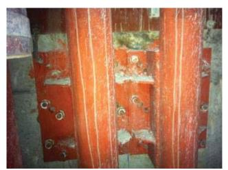
Detail of fixed point designed to be mounted on the wall in shaft lines.
