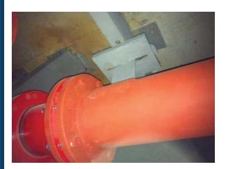
For installations of free floating type system, a sliding rail system should be installed after the fixed point and the expansion joint to prevent deviations from the axis (provided that channel length shall not be shorter than the expansion value).
