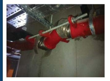
Limit rod nuts should be loosened by 1 nut length after installation.
