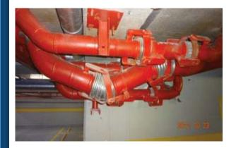
Position single expansion joint on quadruple pipeline without fixed point goes in during testing.
