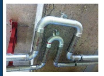
In Omega Flex applications, mounting should be performed between two fixed points like expansion joints.
