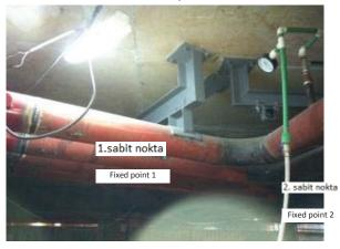
Note that fixed points of expansion joints on heating/cooling lines should NOT be on the same carrier. Expansion joints of heating line and cooling line should be fixed onto different carriers. The system's operation in different modes cause different loads on the main carrier. In such case, moments applied to the different parts of the profile can cause
