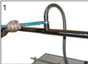
The sprinkler hose's 1" nipple section is attached to the fire line's T or sleeve.
