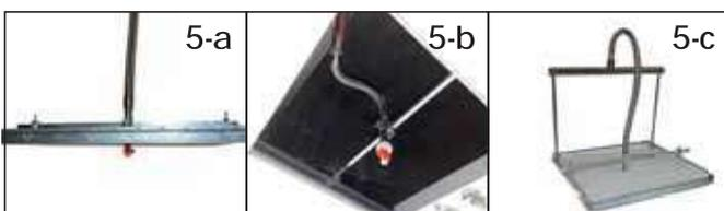
Finally, the hole in the suspended ceiling's middle is centered with the sprinkler hose. The end of the hose should remain at the upper level of the ceiling tile by completely tightening the side supports from the top and sides and clamping them at the center point. The sprinkler nozzle can be repositioned if there is an axial misalignment after installation.
